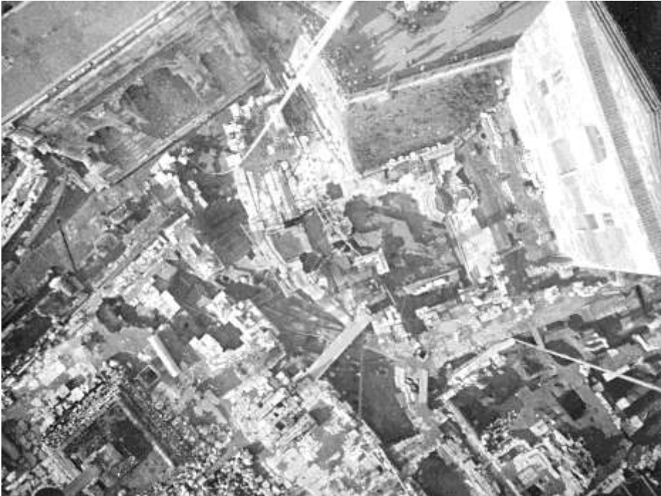
Fig. 2 Excavation campaign in the central part of the Forum (area of Comizio and of Niger Lapis ) recorded by g: Boni on a captive baloon of Brigata Specialisti of the Military Engineers of Italian Army.
